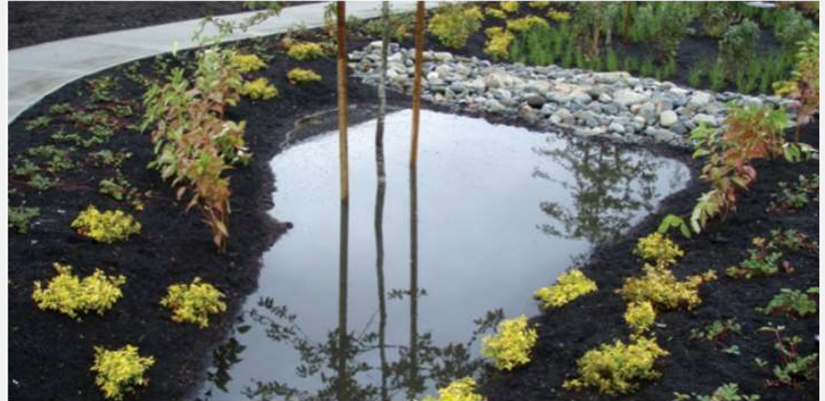
Stormwater Infrastructure Practice - Rain Garden
